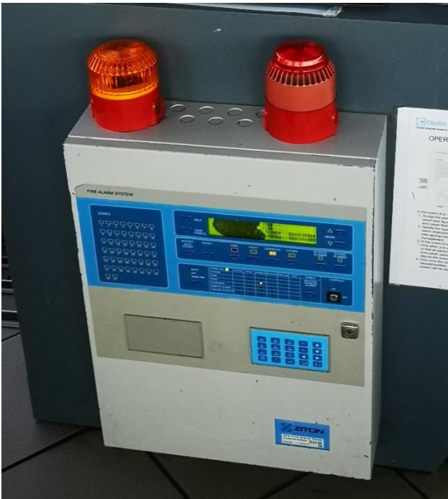
Figure 17. Fire alarm system panel
